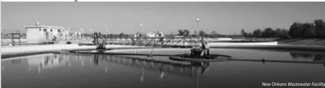
New Orleans Wastewater Facility
